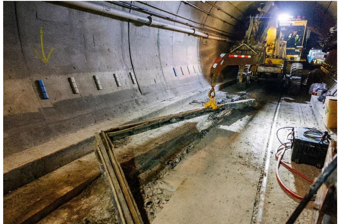
North Bound Rail Replacement in the DSTT – February 2024
